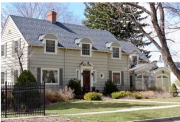
1614 Culebra Place - Broken pediments over the front door, as seen here, are common in Revival styles, rare in Colonial originals. This home also features a unique oculus window by the front door and arched wall dormers.
